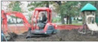
Excavating lead-contaminated soil at playground.
